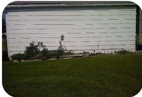
Siding is rotting and needs to be replaced on entire building and Compression on the siding on the north side indicates severe settlement and wall and or floor construction
